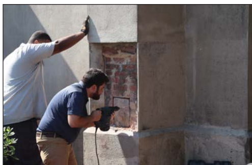
Excavating the cornerstone
